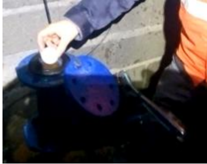
Figure 1 and 2: The ApoleAU In-Line Leak and Pressure Inspection Tool being inserted and extracted into drinking water pipeline
