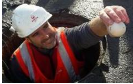
Figure 1 and 2: The ApoleAU In-Line Leak and Pressure Inspection Tool being inserted and extracted into drinking water pipeline
