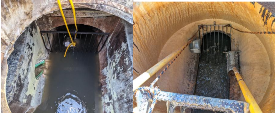
Figure 7 and 8: Typical temporary steel bar screens for device capture (on the left is Richmond and the right is Half Moon Bay).
